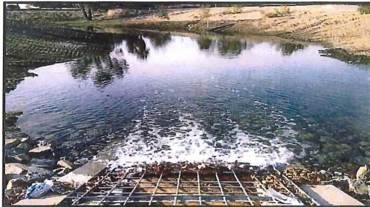
Installed 60-inch connection pipe into Basin 8
