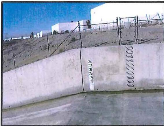
Berm removed and channel cleaned
